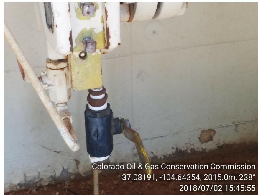
Photo 3. Better view of crack in valve.
