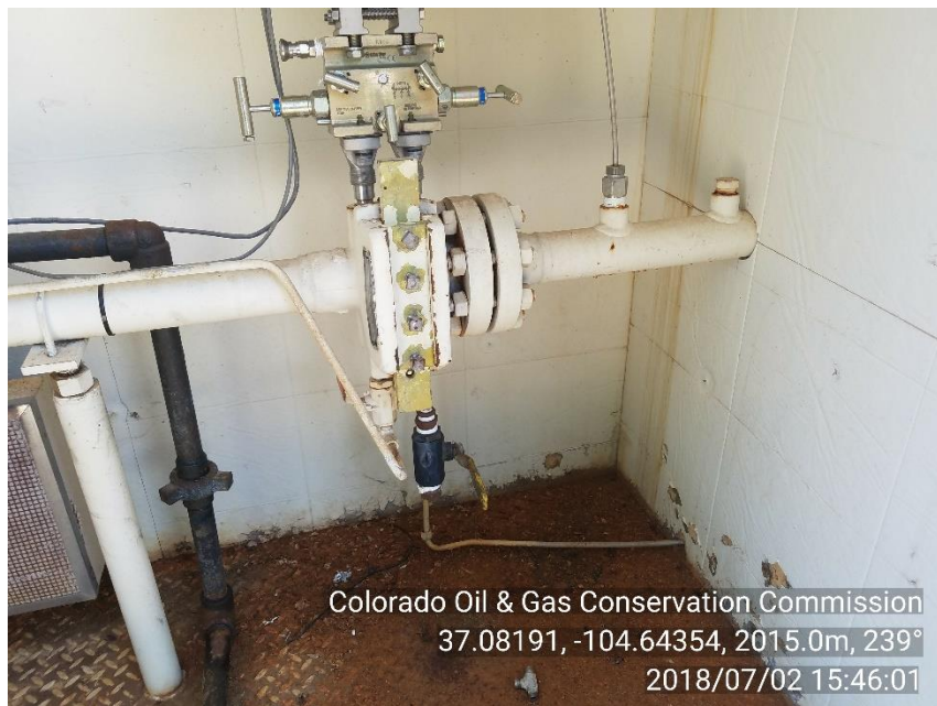
Photo 3. Cracked 1" valve
