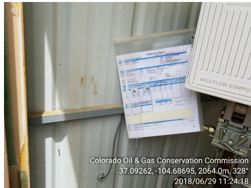
Photo 2. Calibration out of date
