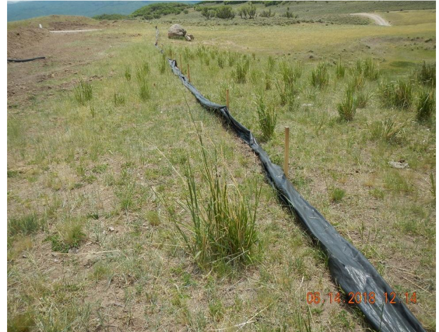
Silt fence in disrepair.
