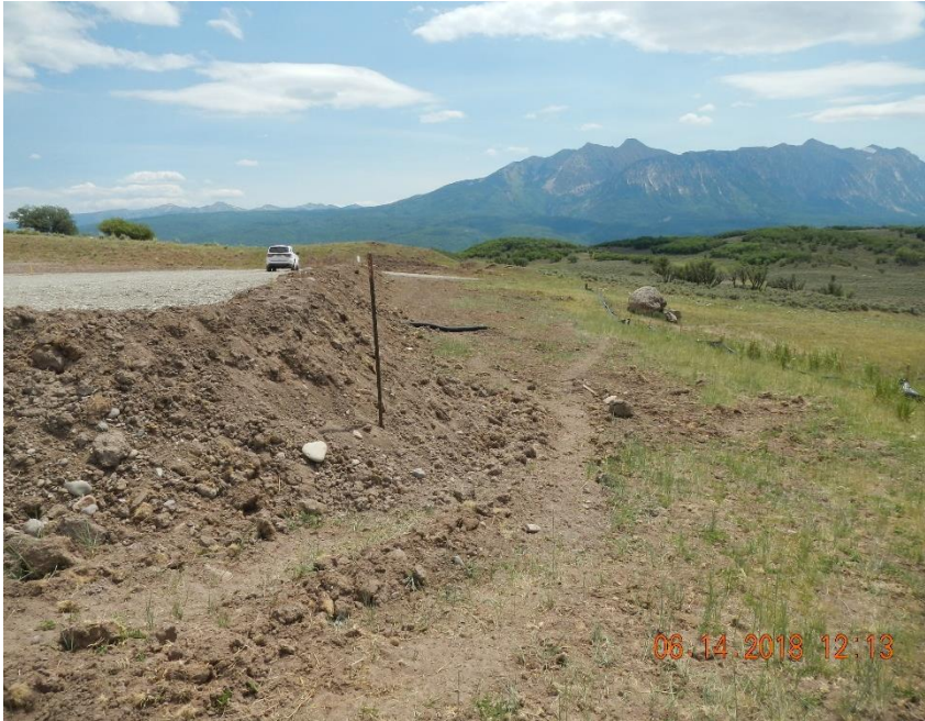
Location berm on southern edge of pad.
