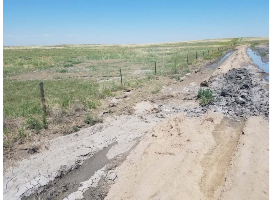
Photo 6 – View of storm water breach and runoff onto State Land Board property to west.
