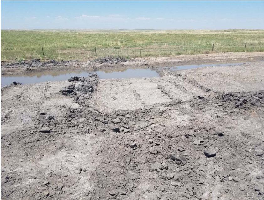
Photo 5 – Area of berm breach and stormwater runoff onto Stand Land Board property to west.
