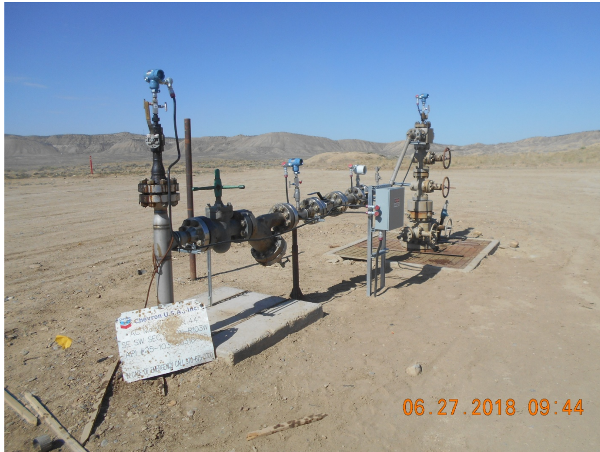
Injection Wellhead
