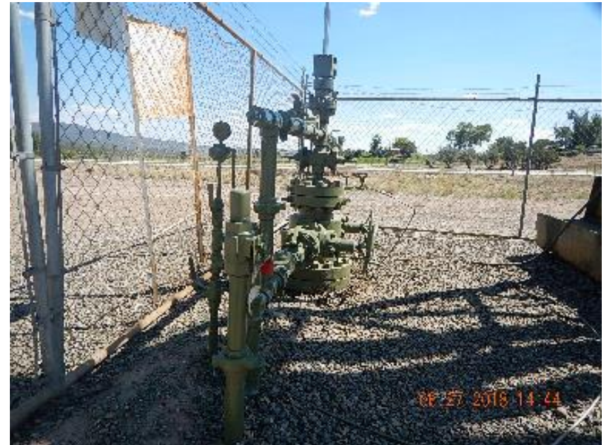
Photo 2: Unused riser at #6-4 wellhead.
