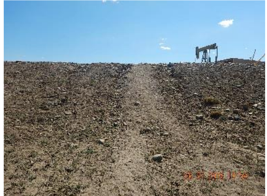
Photo 2: Erosion channels off NE corner fill slope.
