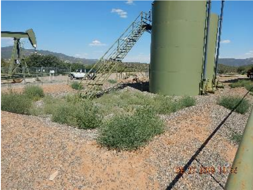
Photo 1: Vegetation growing inside and on tank berms.
