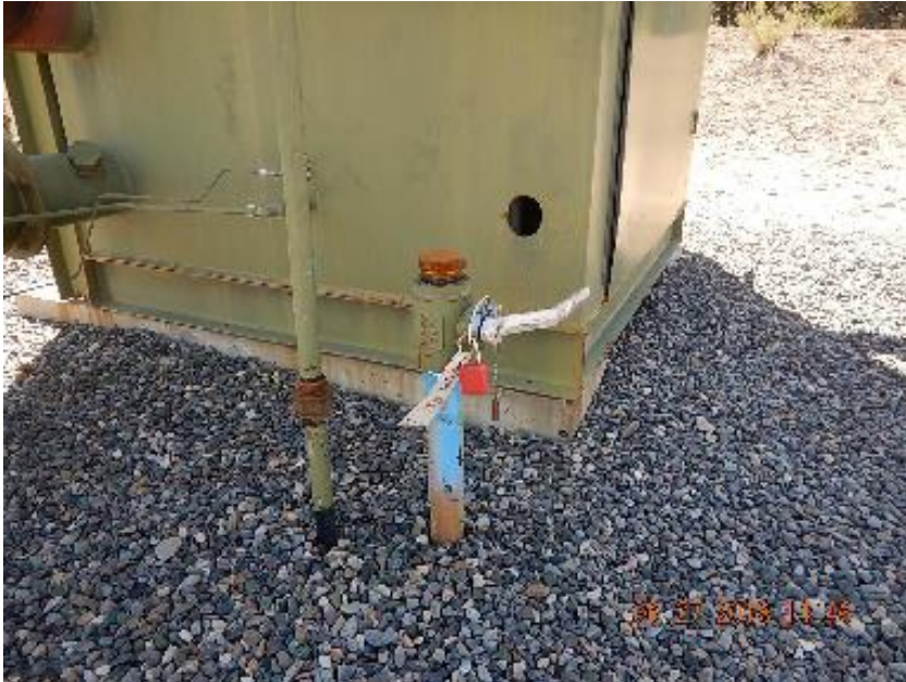
Photo 1: Unused riser at #6-4 separator.
