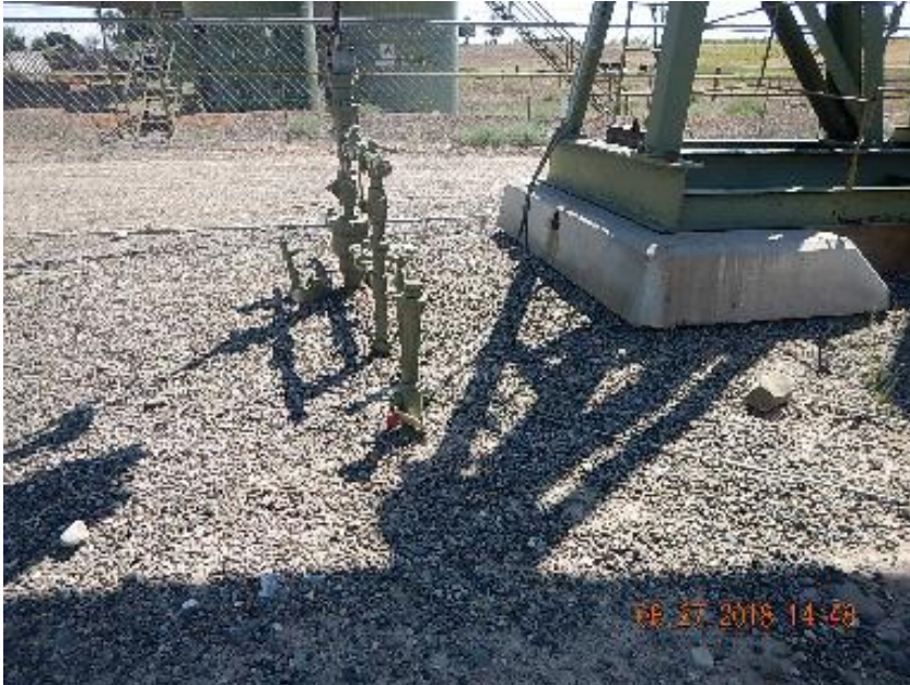
Photo 1: Unused riser at #6-1 wellhead.
