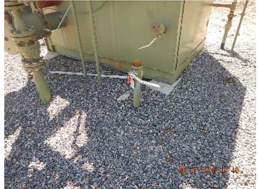
Photo 2: Unused riser at #6-1 separator.
