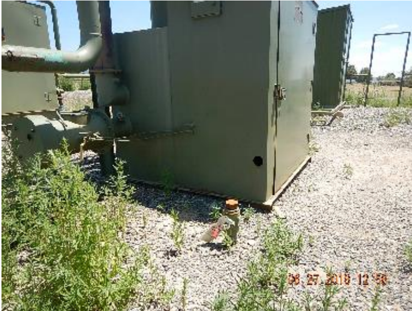
Photo 3: Unused riser at #1-2 separator.
