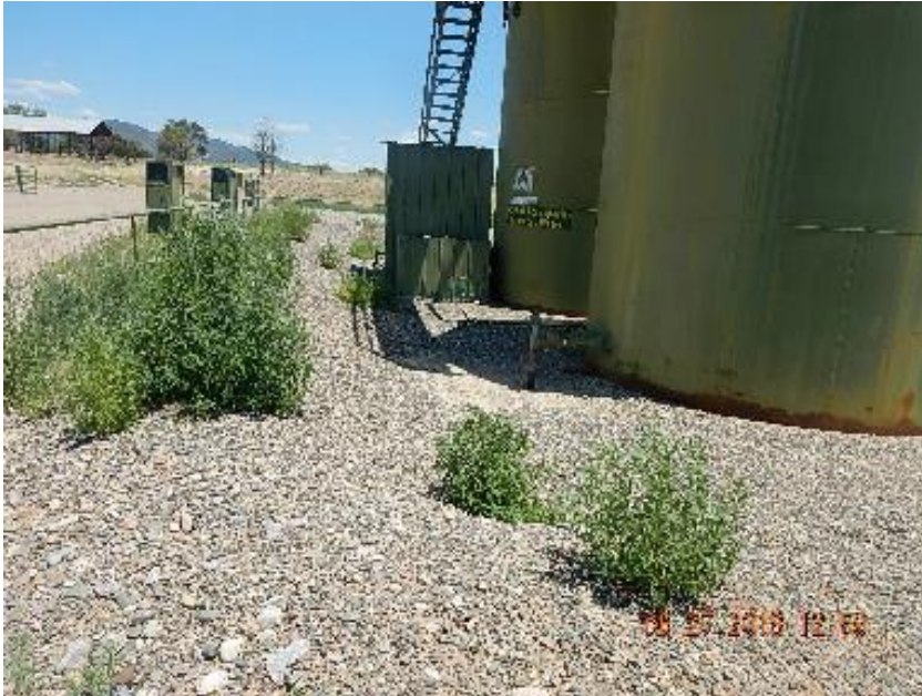
Photo 5: Vegetation growing on and inside tank berms.
