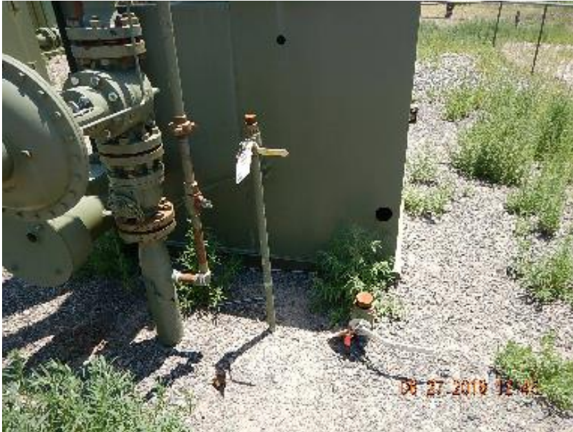
Photo 3: Unused risers at separator.
