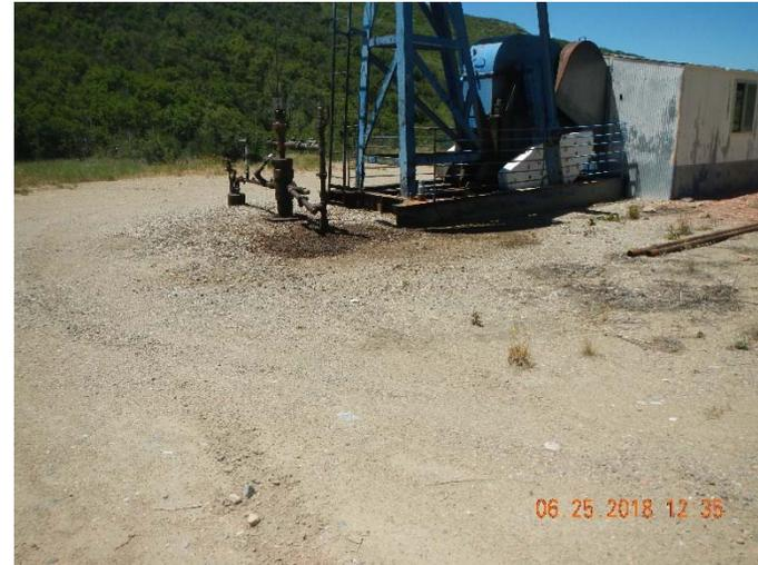
**Photo 2. Stained soil at wellhead.**
