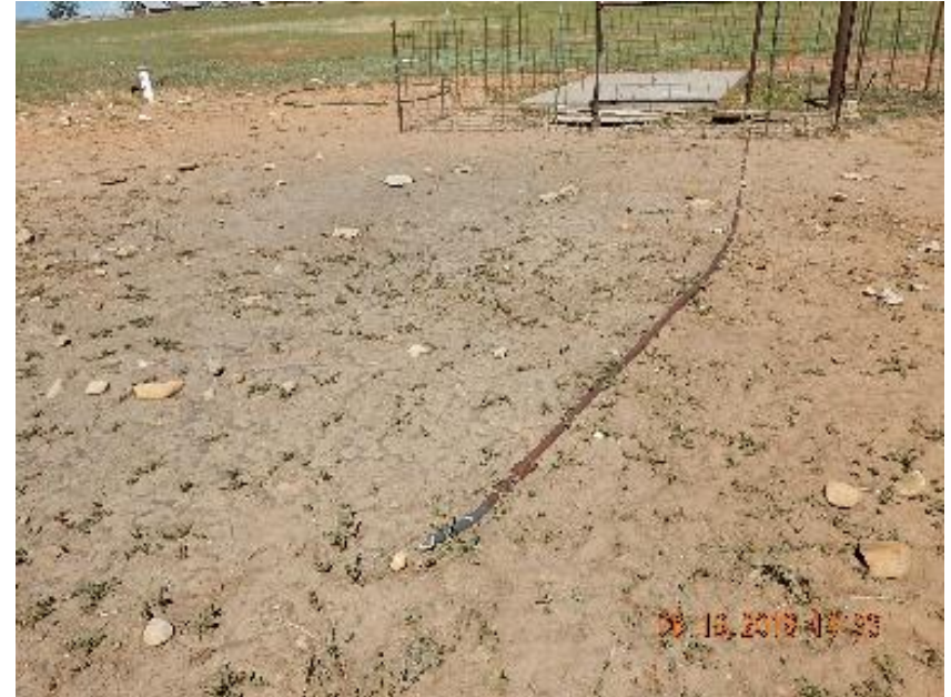
Photo 6: Disconnected steel line.
