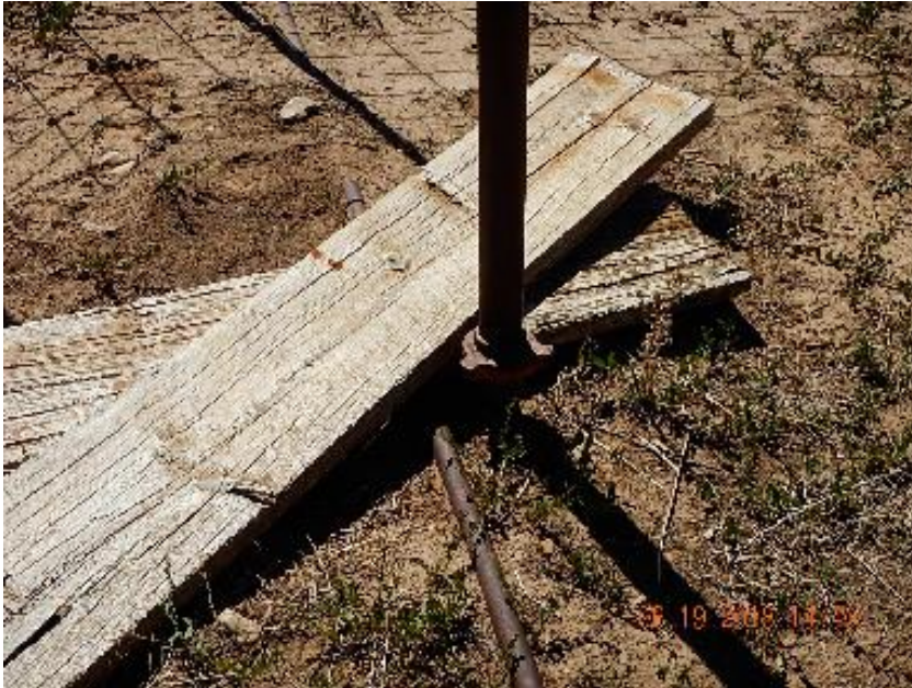
Photo 3: 3" steel flowline from wellhead goes into the ground.
