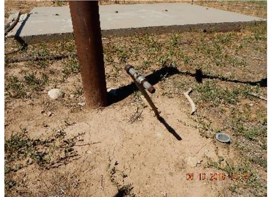
Photo 4: 6" steel riser and 1" steel riser at wellhead.
