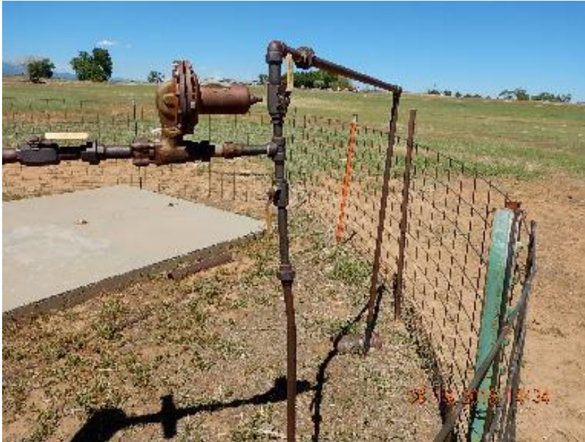
Photo 5: 1" steel line from 6" riser to regulator and split into (2) 1" lines that go into ground.
