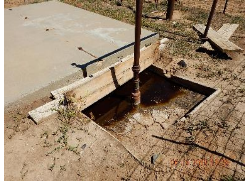
Photo 2: Wellhead cellar with standing fluids.
