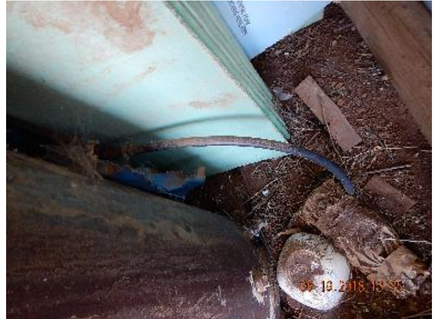
Photo 8: Flow line out of dryer tank connecting to black poly line.
