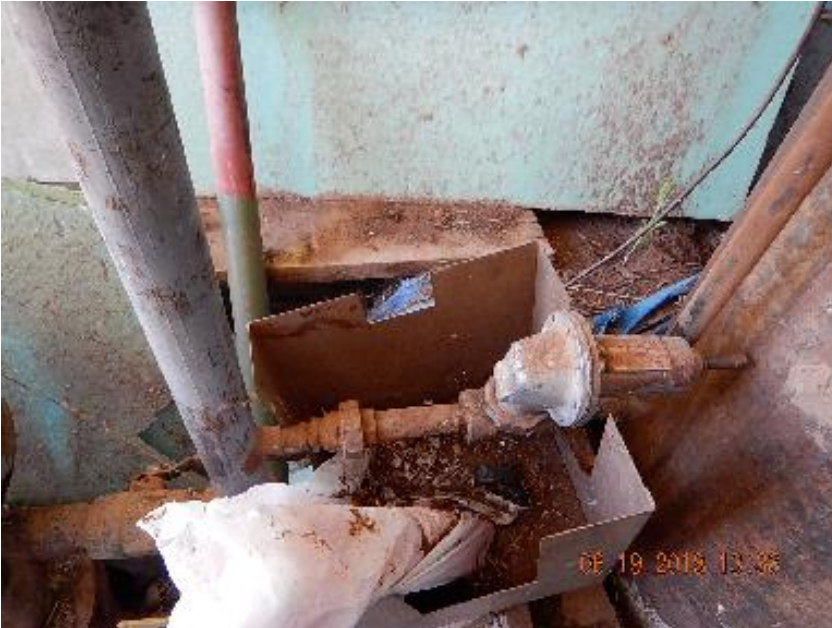
Photo 7: Flow line from wellhead casing to dryer tank.
