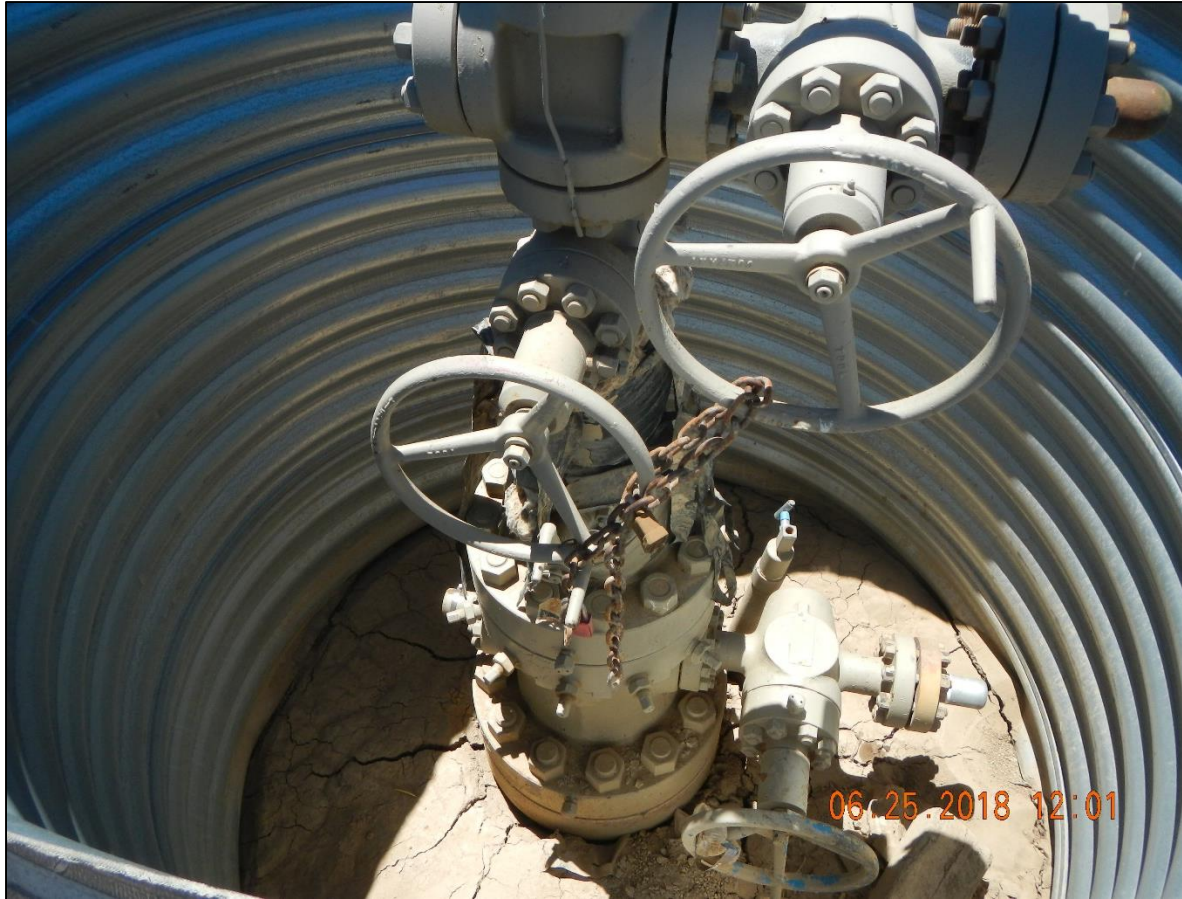
Temporary abandoned well. No well sign.
