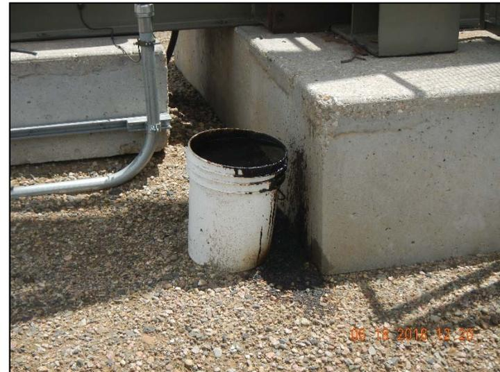
**Photo 2. Overflowing bucket at pump jack base.**
