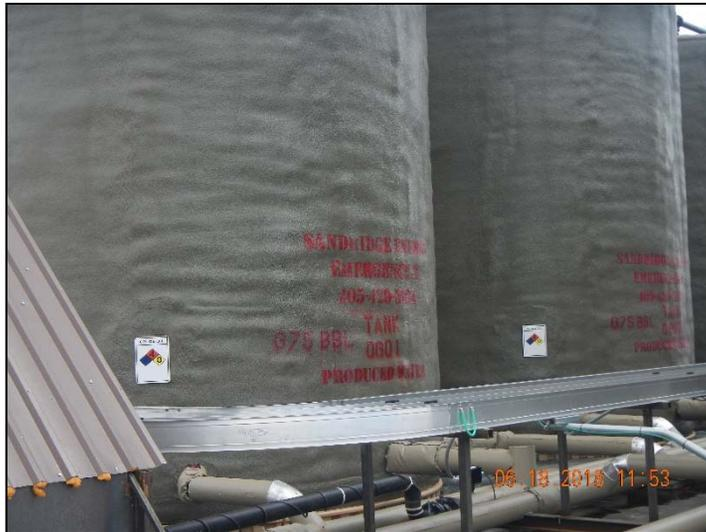
Photo 3. Crude Oil NFPA diamond on tank labeled Produced Water.
