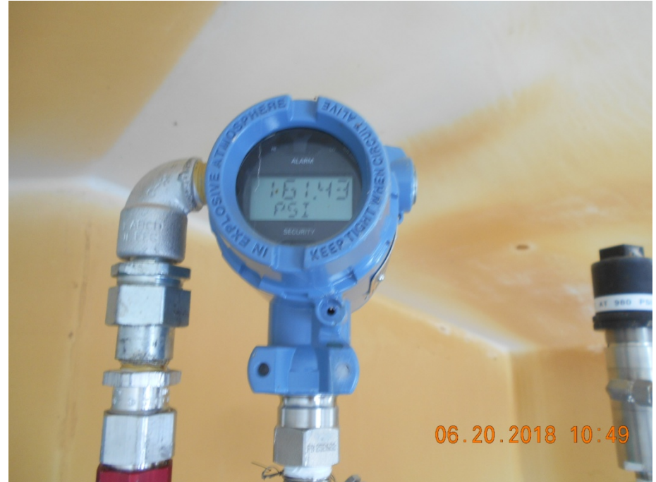
Injection wellhead tubing gauge
