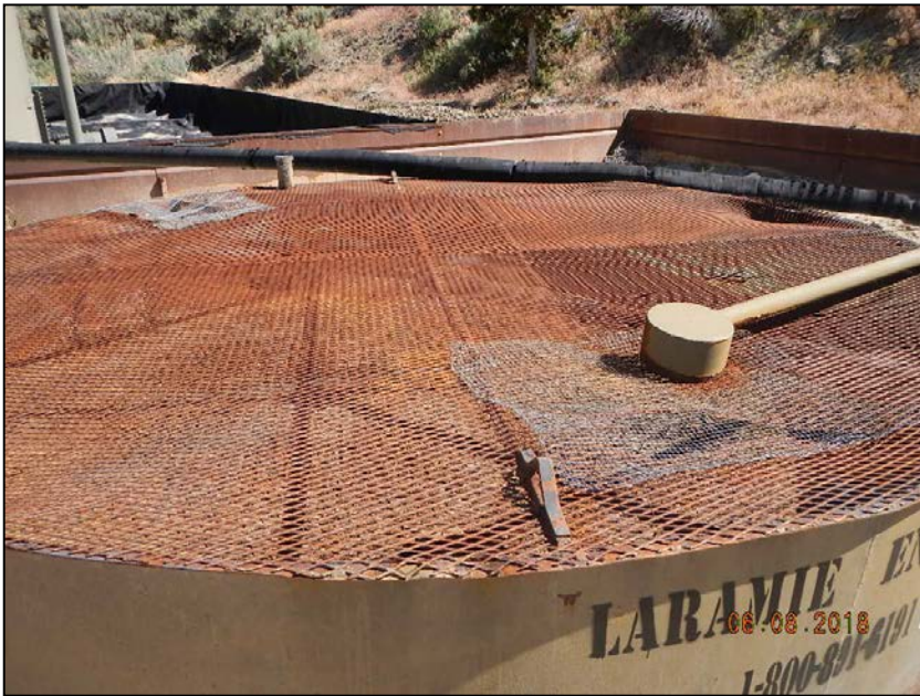
Photo 1. Bird protection repaired.
