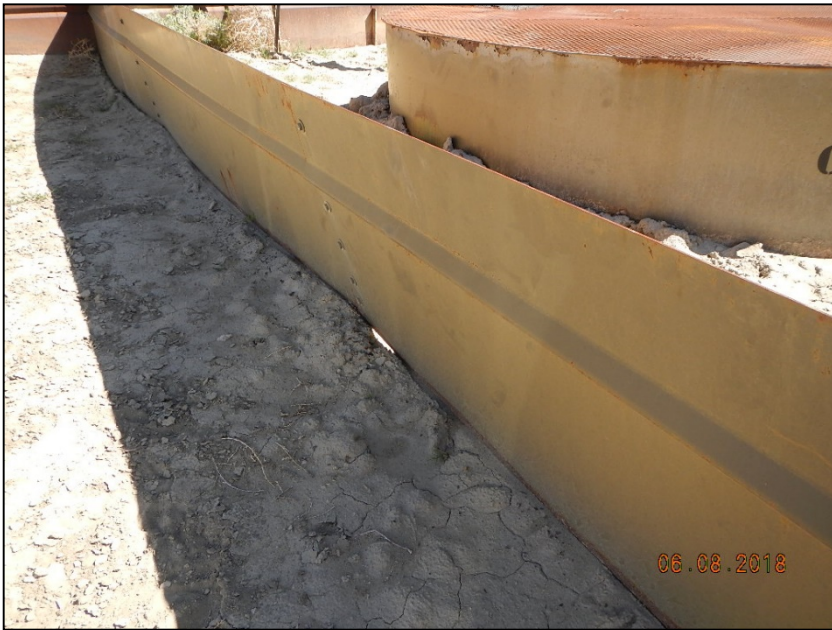
Photo 3. Berm has not been repaired. Original corrective action and date still apply.
