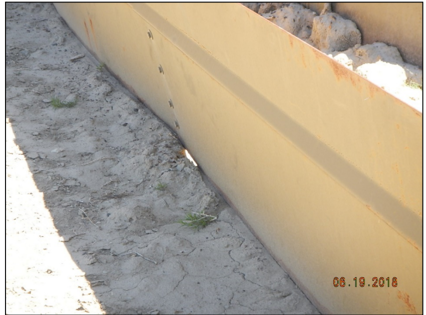
Photo 2. Gap under containment still exists. This is the third inspection with this CA.
