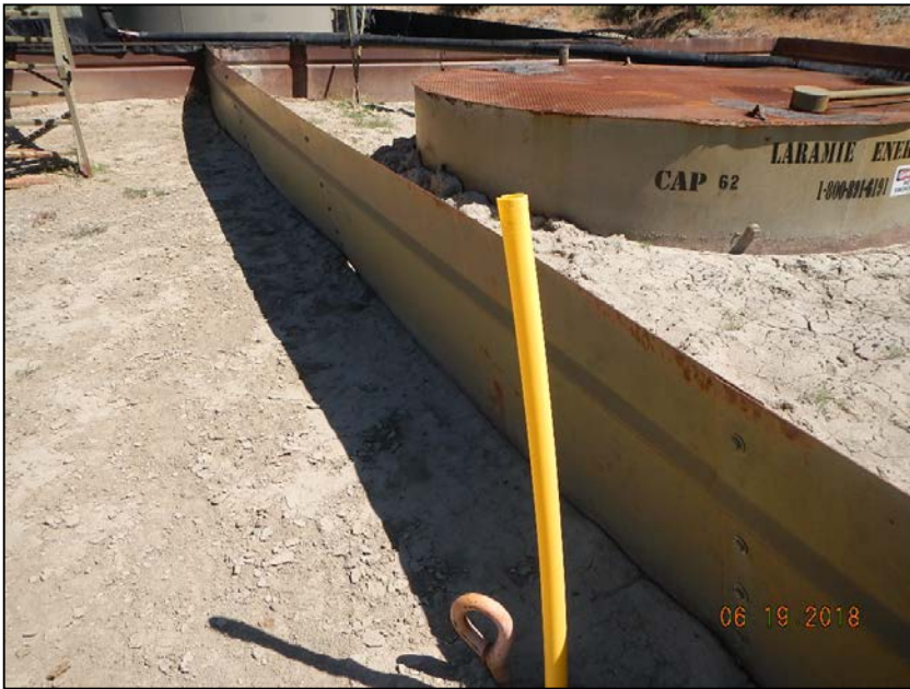
Photo 1. Gap under containment still exists. This is the third inspection with this CA.
