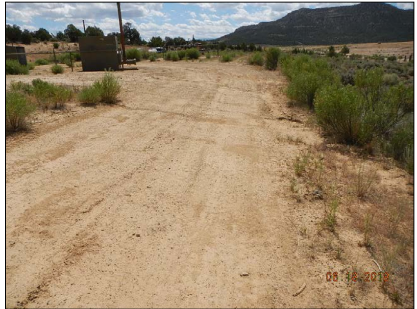
Photo 2. Erosion across access road.
