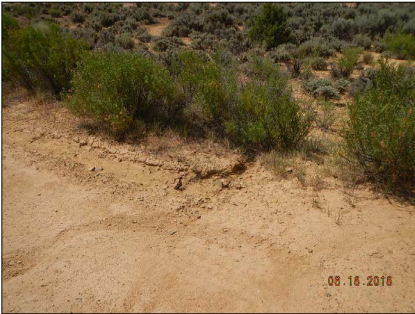
Photo 3. Erosion across access road.
