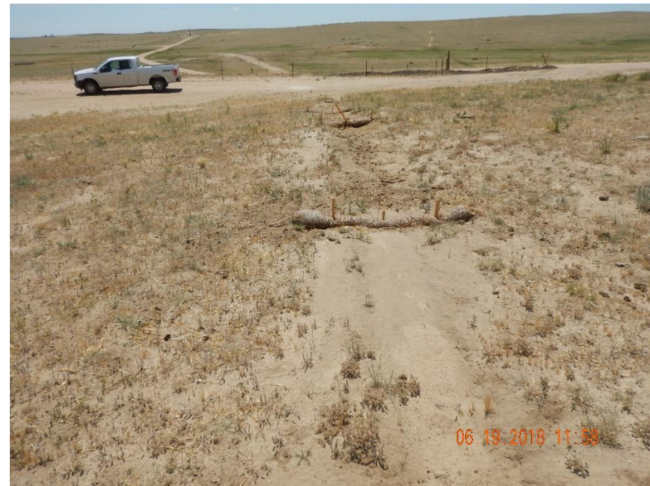
Photo 2: Photo taken from the northwest end of the location, facing south. Photo shows straw wattles have been installed on the north end. Wattles do not appear to be in proper functioning conduction, or have filled with sediment.
