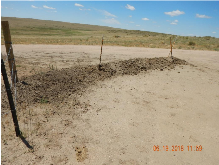
Photo 3: Photo taken from the west end of the location. Photo shows water bar. BMP does not appear to have been installed in accordance to good engineering practices; water bar has not been consolidated or in proper functioning conduction, and is considered a sediment source.
