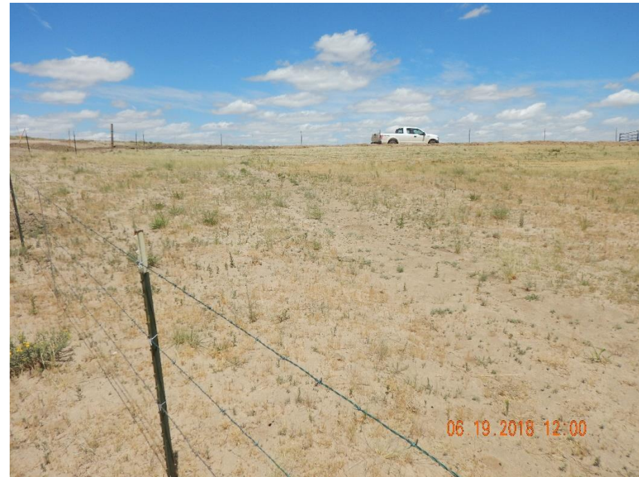
Photo 6: Photo taken from the south end of the location, facing north. Photo shows interim area has been fenced and slope has been repaired and stabilized with straw blankets.
