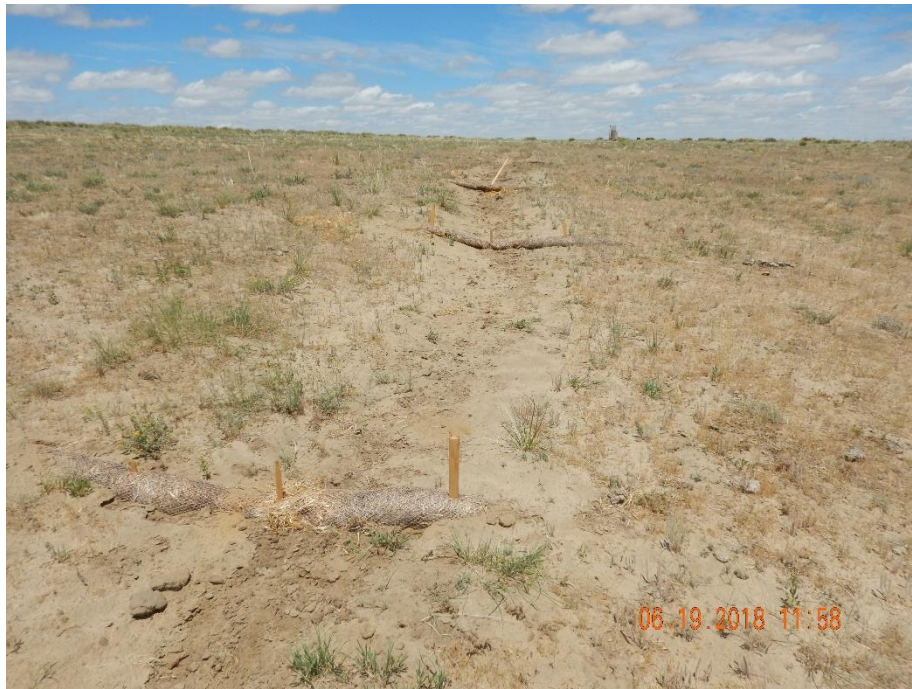
Photo 1: Photo taken from the northwest end of the location, facing north. Photo shows straw wattles have been installed on the north end. Wattles do not appear to be in proper functioning conduction, or have filled with sediment.
