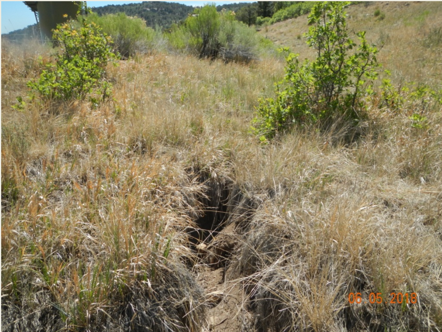
Photo 4. View of erosional channel and tunneling in the southwestern project area, where concentrated stormwater flows down a diversion from the southern edge of the well pad. Photo is facing upstream toward the well pad.
