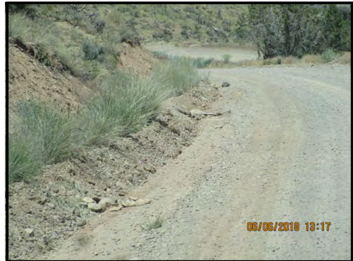
Bar Ditch Re-defined, rock check dams installed to slow water velocity
