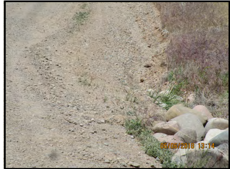
Bar ditch re-defined on east side, looking down the acc. rd from pad
