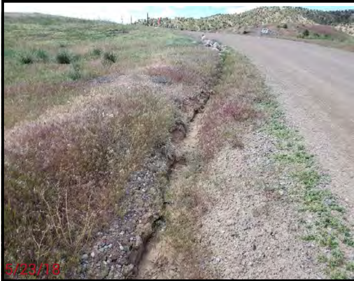
Ditch erosion along side of road on east side
