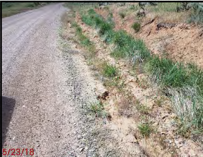
Ditch erosion along side of road on east side. Looking down hill
