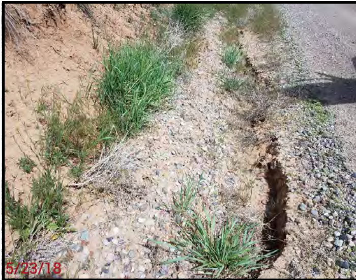
Ditch erosion along side of road on West side. Looking down hill
