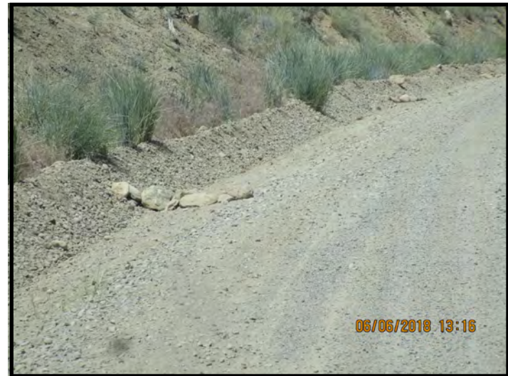
Bar Ditch Re-defined, rock check dams installed to slow water velocity
