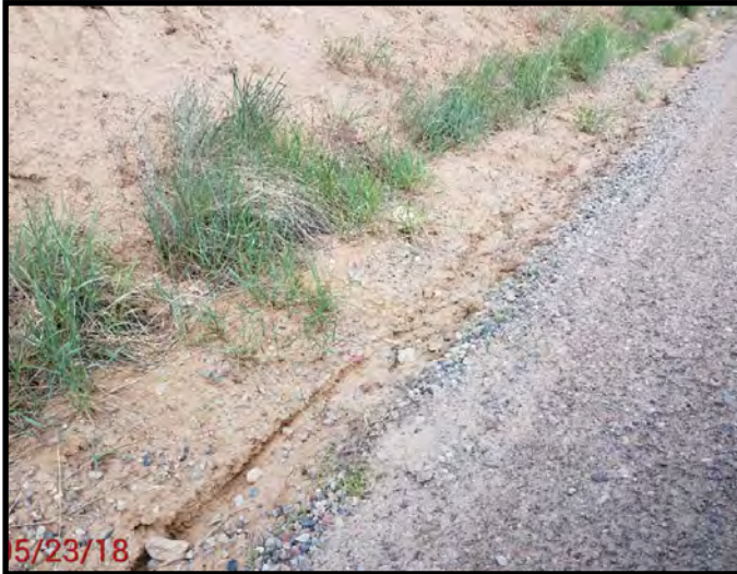
Ditch erosion along side of road on east side near curve
