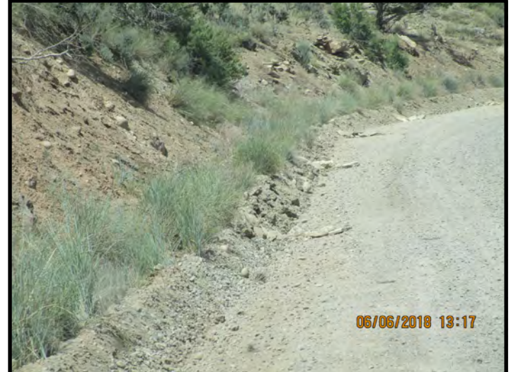
Bar ditch re-defined/check dams in place
