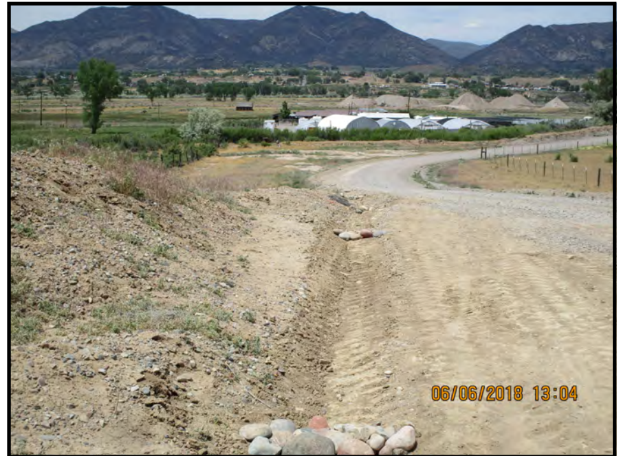
Bar Ditch re-defined, rock check dams installed
