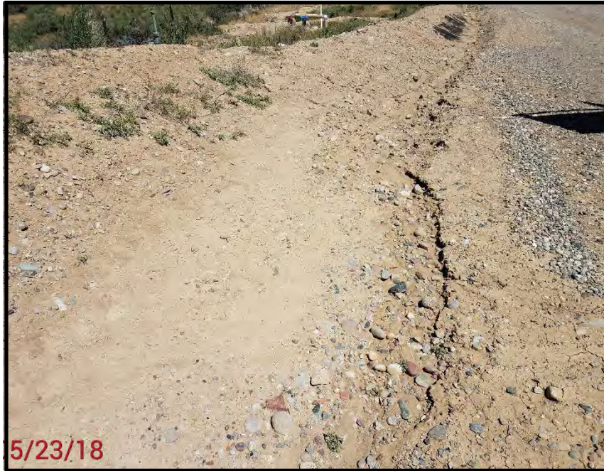
Erosion along West side of access road
