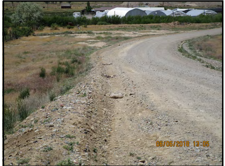
Bar Ditch re-defined, rock check dams installed
