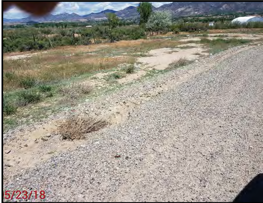
Erosion along West side of access road
