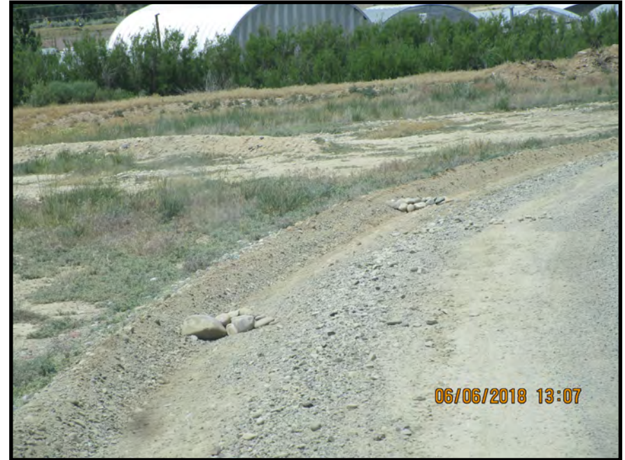
Bar Ditch re-defined, rock check dams installed
