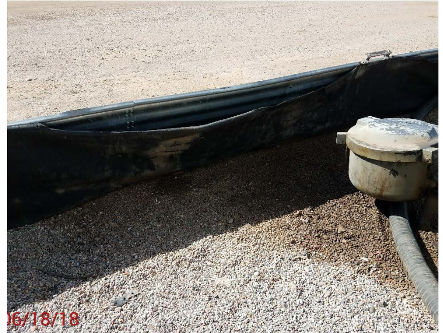
Location Photo #12, Liner falling down
