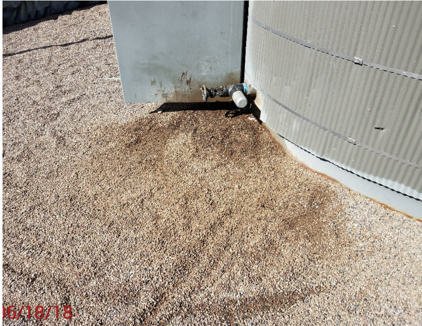
Location Photo #15, Stained Material in Tank Containment
