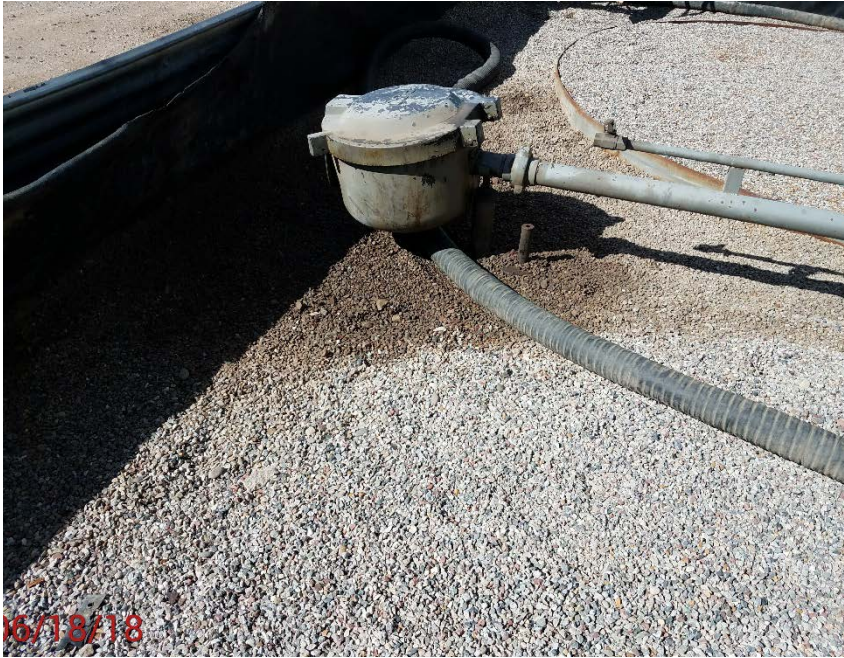
Location Photo #7, Stained Material in Tank Containment
