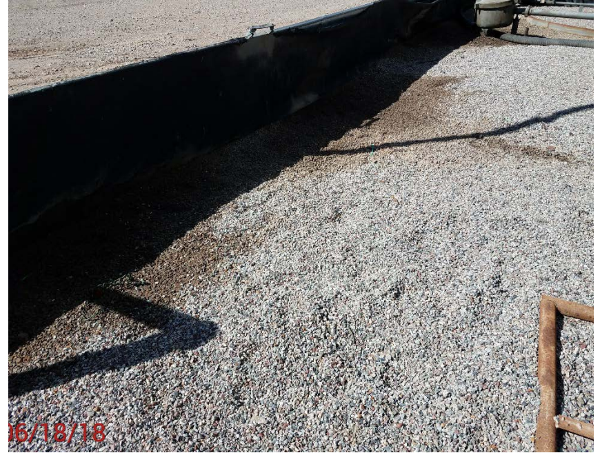
Location Photo #6, Stained Material in Tank Containment
