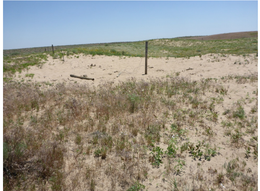
Photo 4. Photo taken from the south end of the location, facing East. There is a fenced in pit area remaining on location that will need to be re-contoured and re-graded. See comments from Photo 2.
