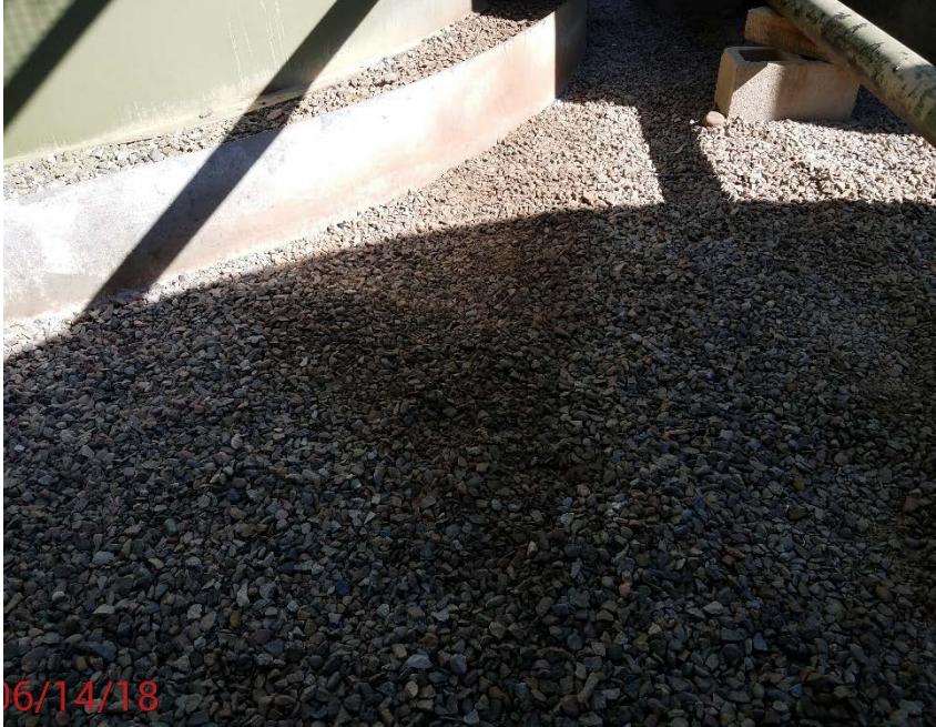
Location Photo #7, Stained rock in battery containment
