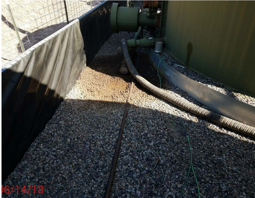
Location Photo #5, Stained rock in battery containment
