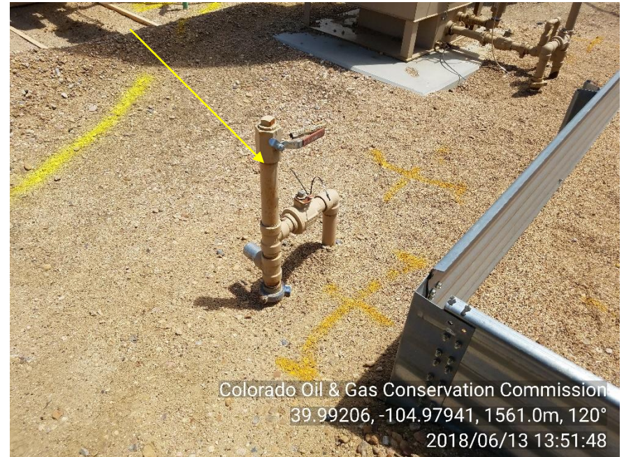
Photo 4. Unused unmarked riser
