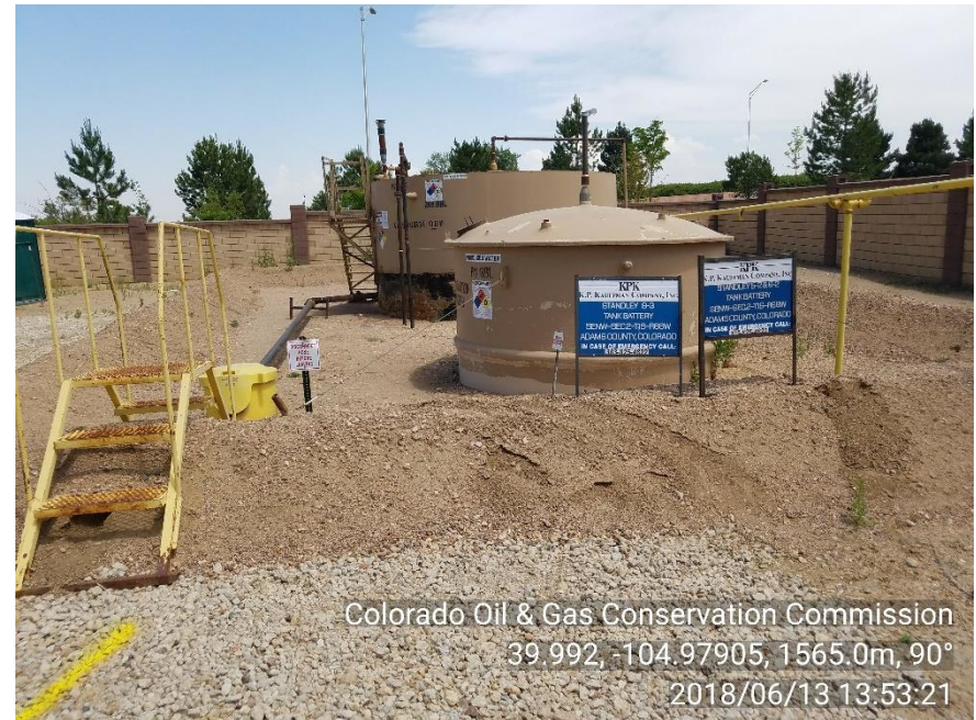
Photo 2. Tank battery
