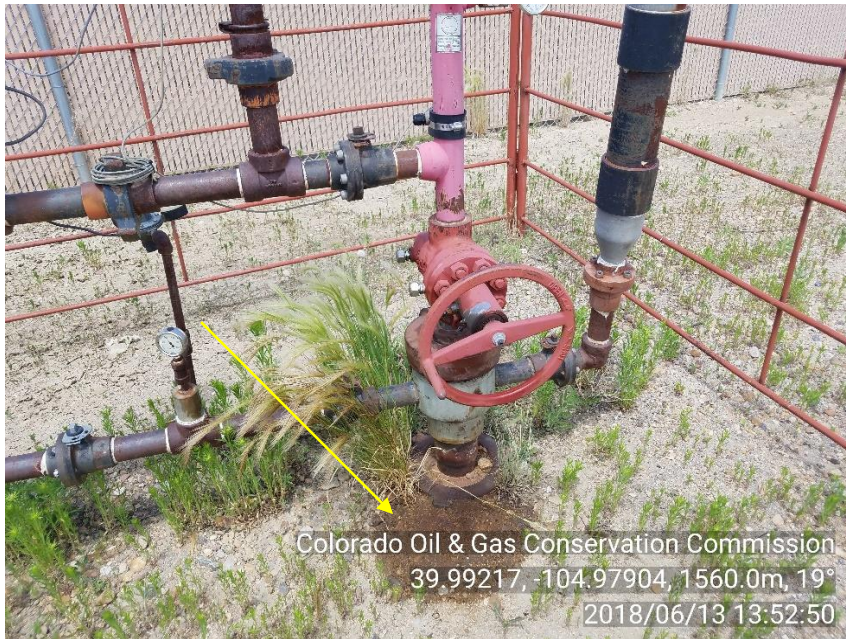
Photo 3. Stained soil around #6-2 wellhead
