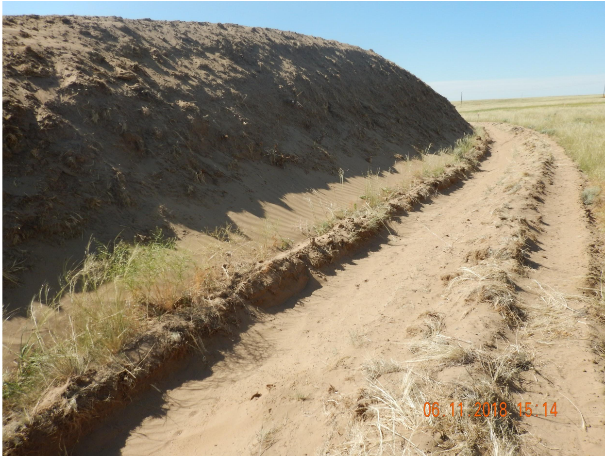
Photo 7. Photo taken from the northeastern perimeter of the location, facing North. Topsoil has been salvaged and stored along the northeastern location but has not been properly stabilized. The ditch BMP is filling in from unconsolidated material.
