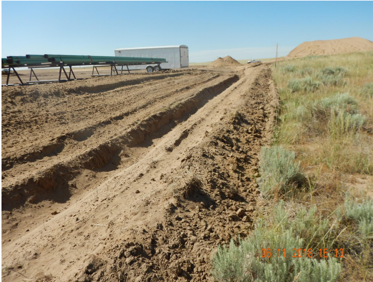
Photo 6. Photo taken from the southeastern perimeter of the location, facing North. See comments under Photo 1. Portions of the ditch BMP appear to be filling in from unconsolidated material.
