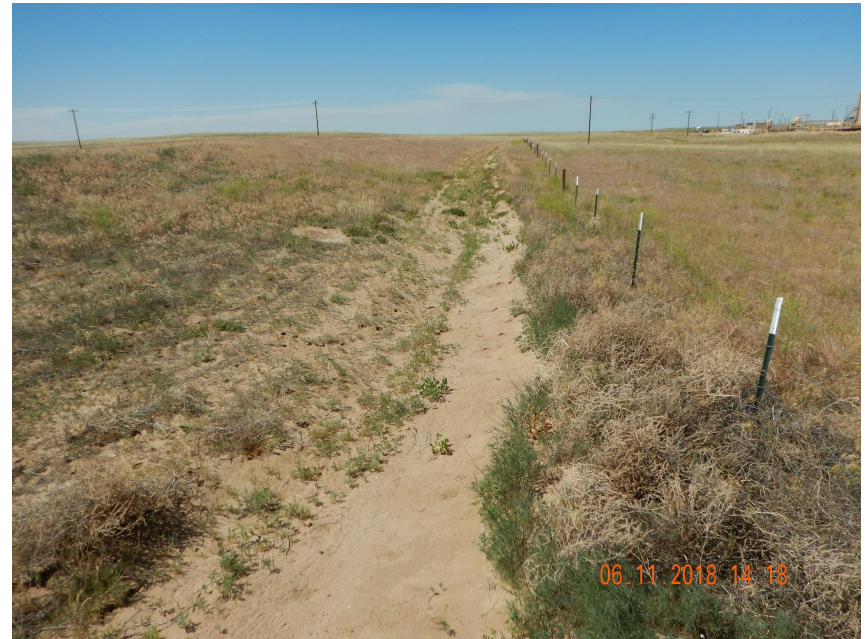
Photo 8. Photo taken from the southeast perimeter of the location, facing North. See comments under Photo 5. Note- a ditch and berm BMP has been installed around the southern and eastern perimeter of the location.
