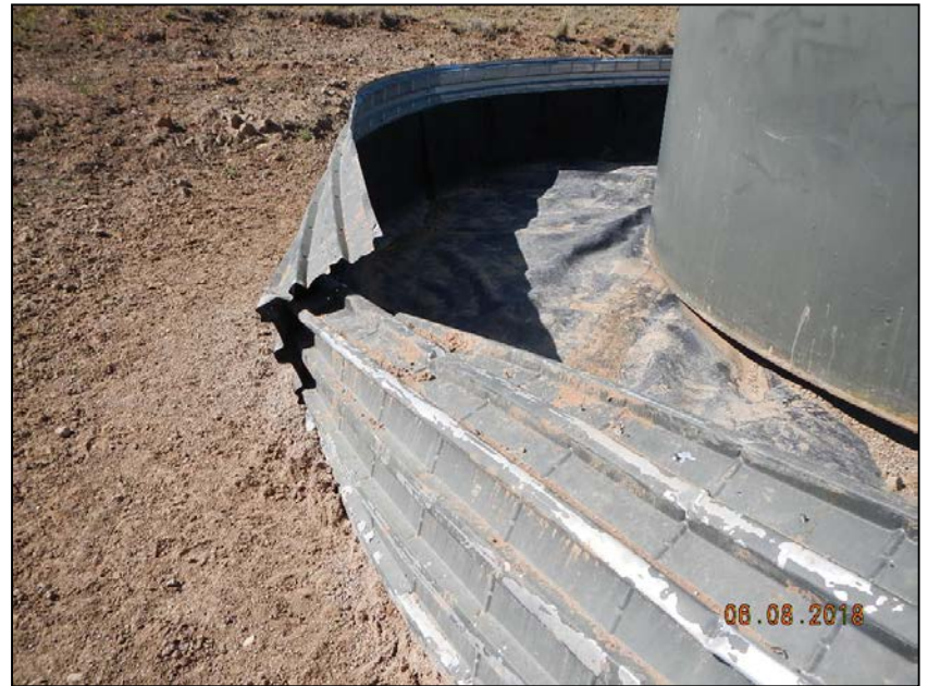
Photo 2. Damaged containment.
