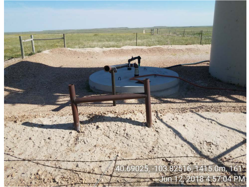
Photo 3: No contents, capacity, NFPA labeling for concrete vault.
