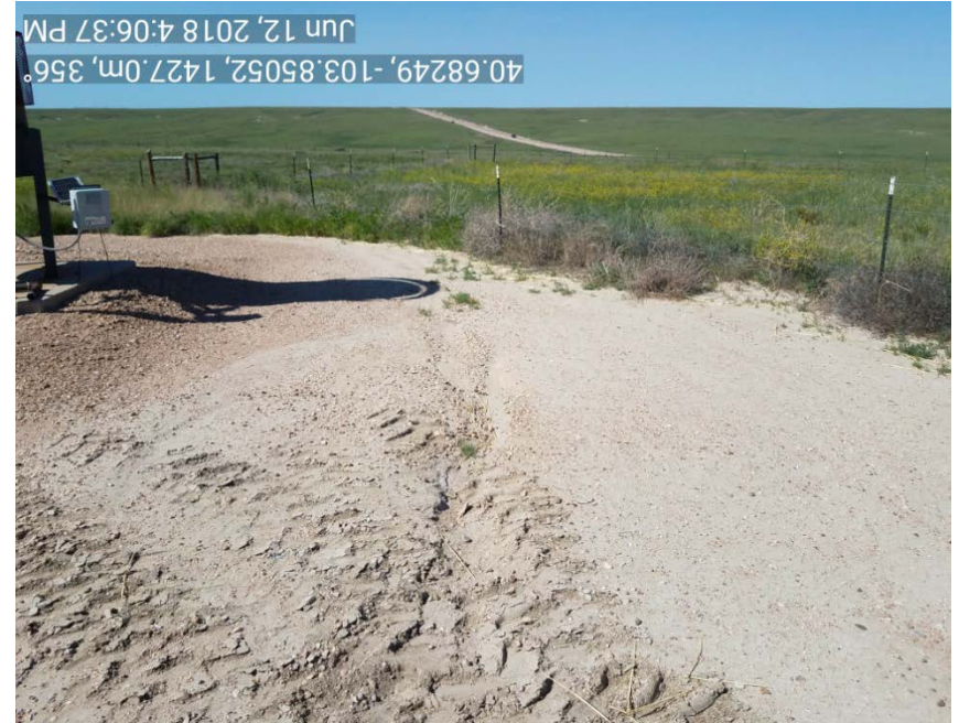
Photo 3: Stormwater erosion on NE corner of location
