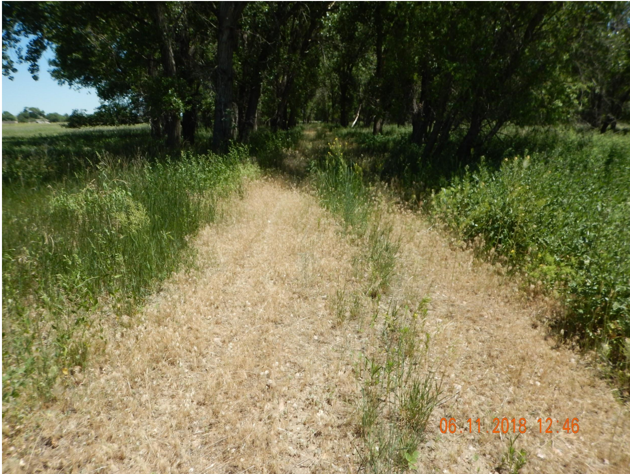
Photo 1. Photo taken from the start of the access road, facing East. Access road is evident and does not meet Rule 1004 standards. Access road appears to be compacted with undesirable vegetation, including noxious weeds (Canada and Musk Thistle).
