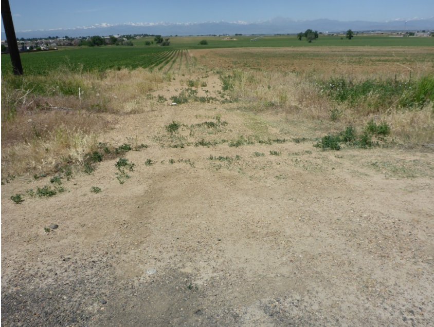
Photo 1. Photo taken from the access road looking towards the location, facing West. The gravel has not been removed and compaction has not been alleviated along the first part of the access road.
