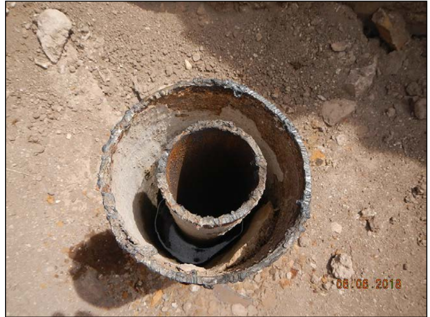
Photo 4. Cut off casing.
