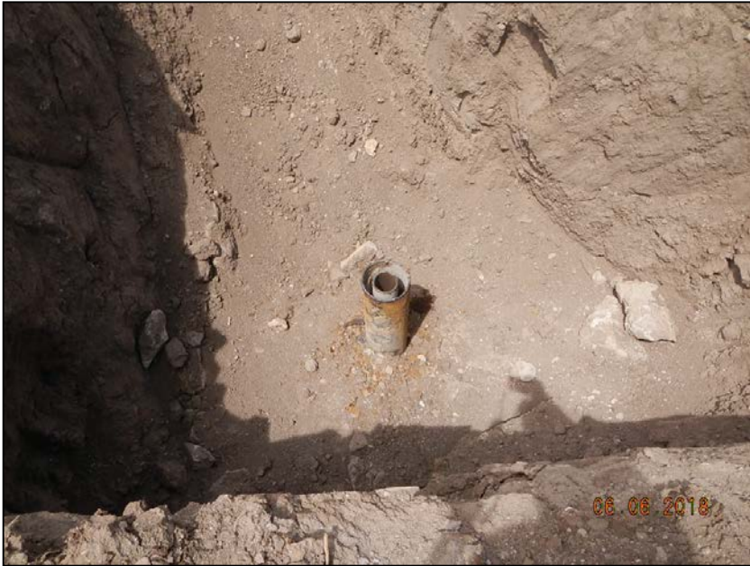
Photo 3. Cut off casing.
