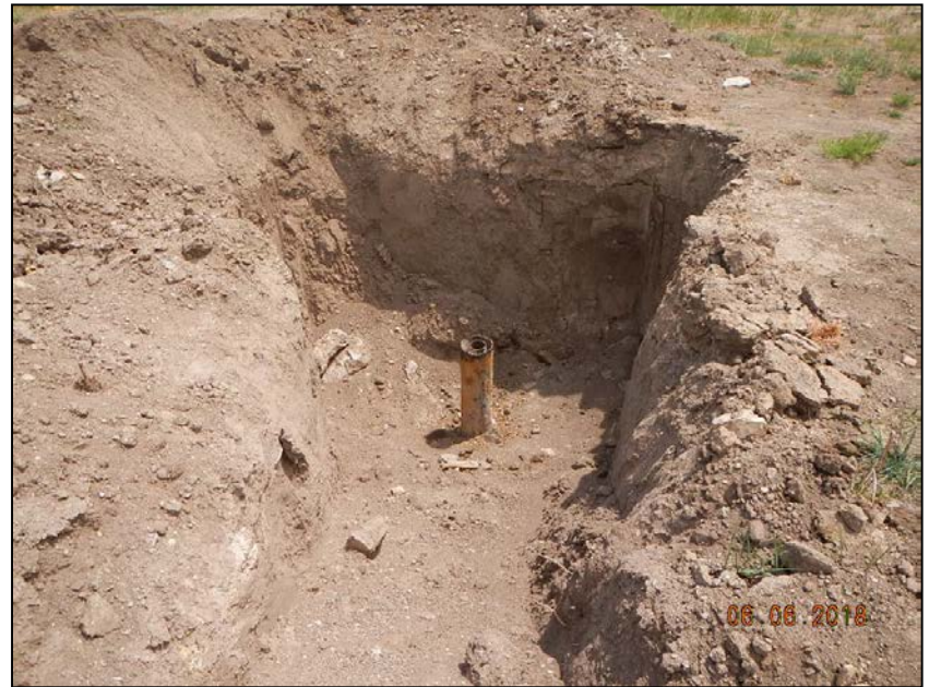
Photo 2. Cut off casing.
