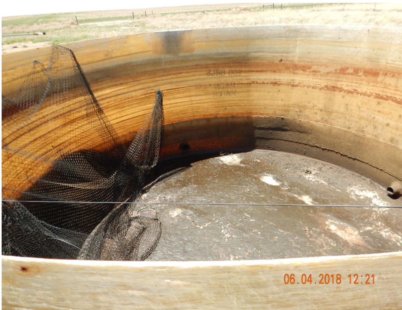
Netting on open tanks inadequate. Wildlife protection devices not adequate
