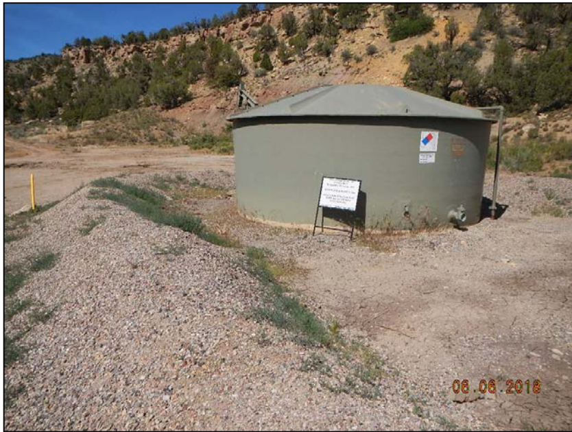
Photo 1. Vegetation still present in tank containment and on berm.
