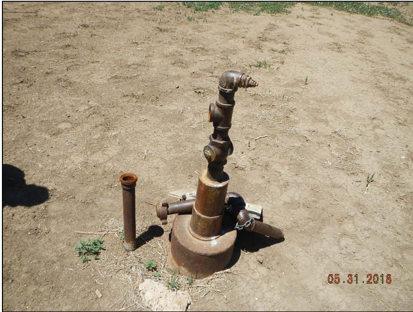
Wellhead and wedge valve with disconnected flowline segment and flowline riser
