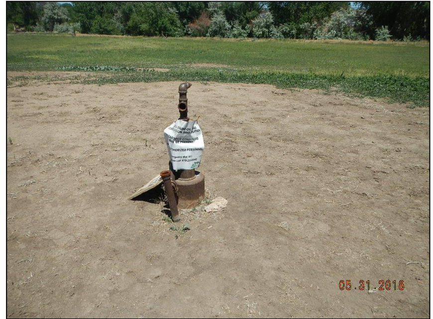
Wellhead with COGCC investigation sign installed, note circular area void of vegetation around well
