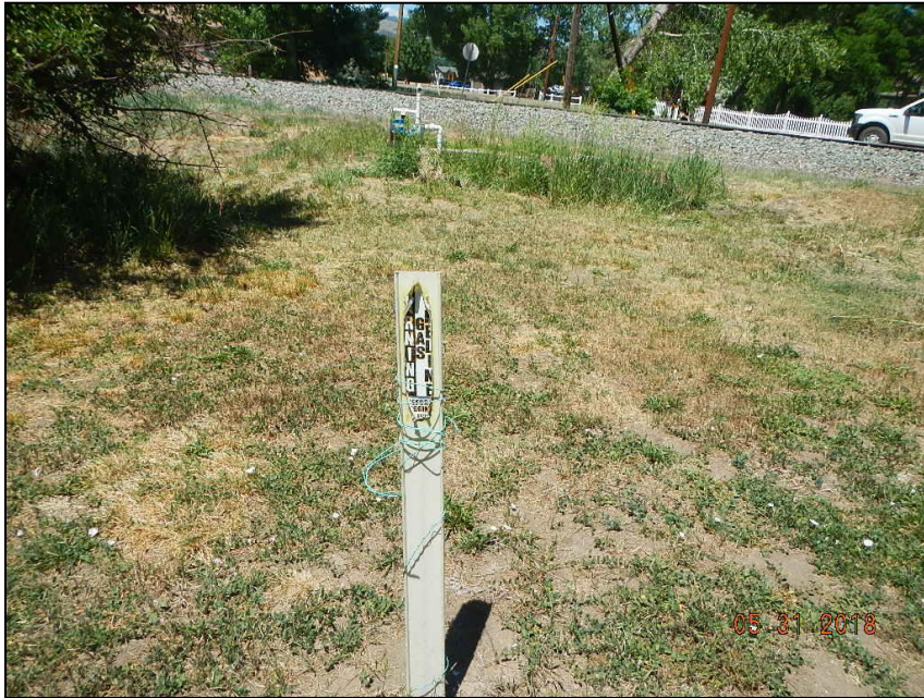
Inadequate flowline marker as line goes north under RR tracks
