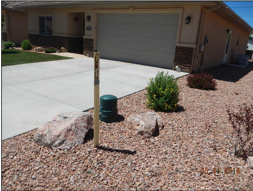
Inadequate flowline marker as line goes through property and near home
