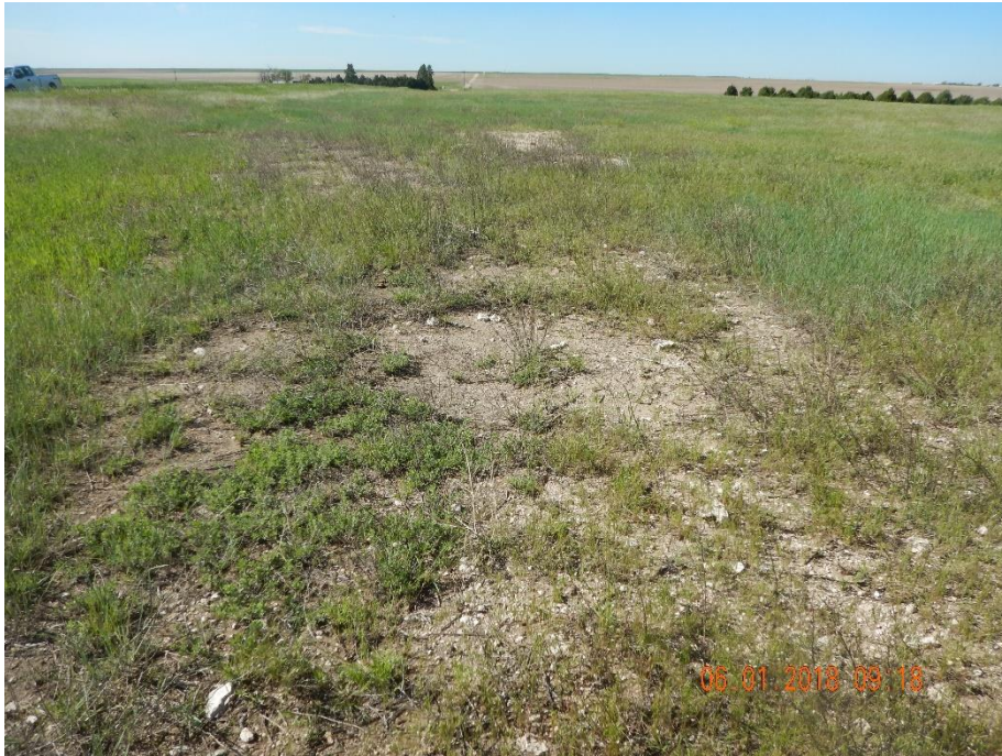
Photo 1: Photo taken from the northeast end of the pit location, facing south. Photo shows areas of the pit remain predominantly bare and exposed soil. Vegetation seen in photo largely undesirable weedy plant species such as cheat grass. Unable to find evidence that additional reclamation activities have been conducted in accordance to reclamation requirements and standards, or per corrective actions.
