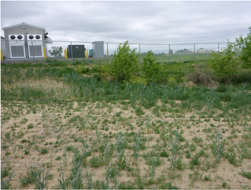
Photo 5. Photo taken from the facility location, facing Southeast. Appears the Operator has performed final reclamation activities on the facility location, with the evidence of drilling rows, straw crimped mulch. See comments under Photo 1.
