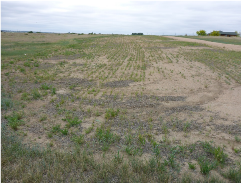
Photo 1. Photo taken from the location entrance, facing North showing the facility location. Appears the Operator has performed final reclamation activities, with the evidence of drilling rows, straw crimped mulch, and perennial grass starting to come in.
