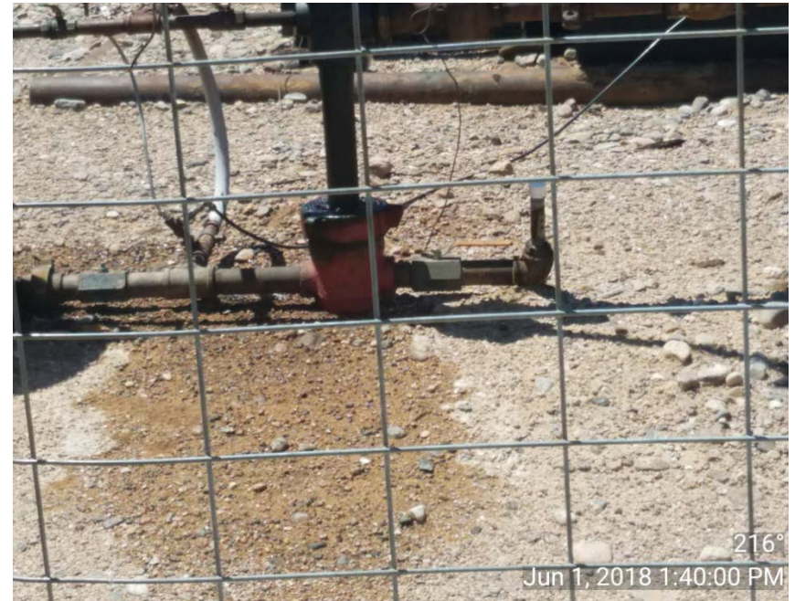
Photo 2: Stained soil at wellhead
