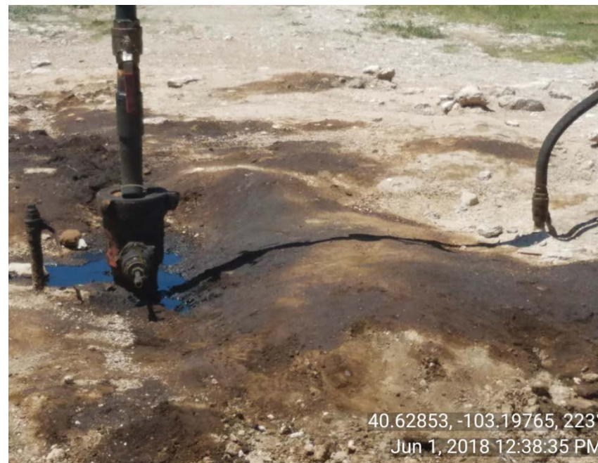
Photo 2: Stained soil at wellhead, free hydrocarbons
