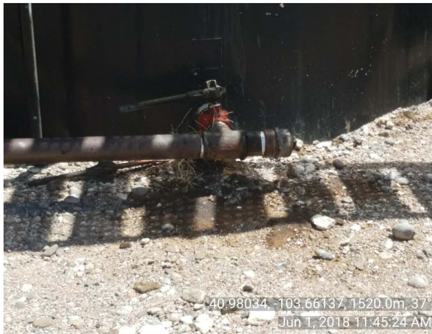
Photo 6: Stained soil at fitting
