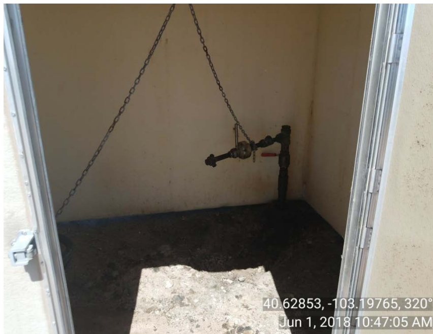
Photo 1: Wellhead, currently TA.
