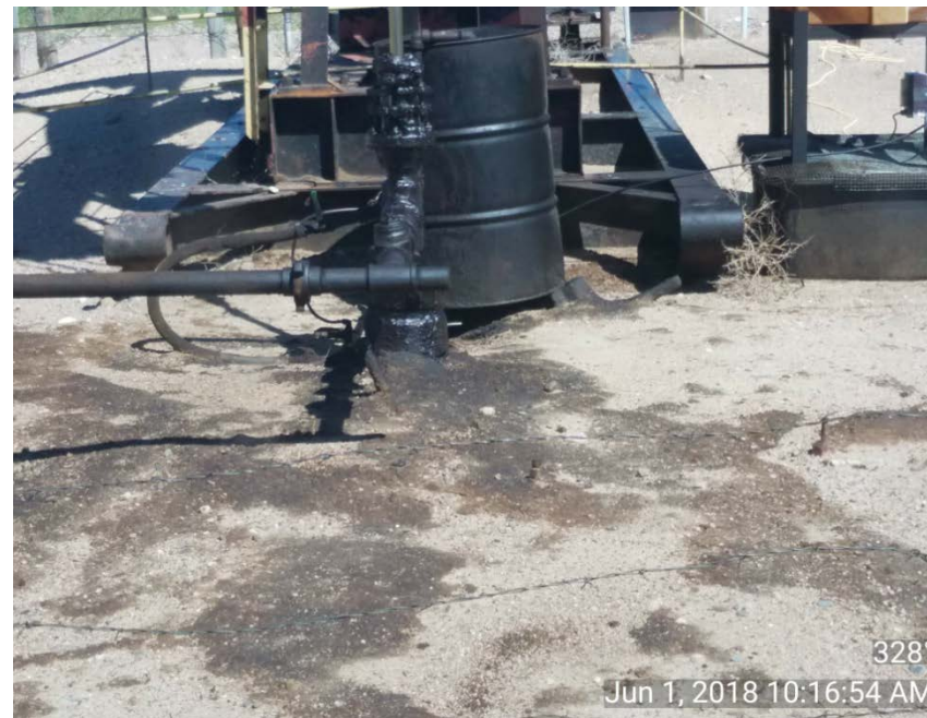
Photo 2: Stained soil at wellhead
