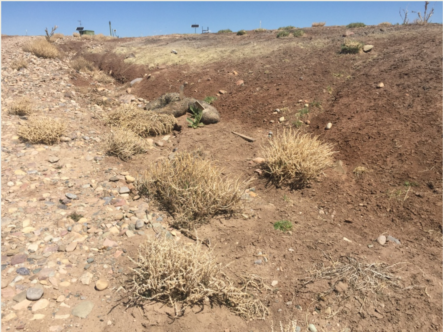
Photo 5. View of wattles no longer functioning and insufficient, and eroding channel along northeastern edge of the access road. Slope above channel is not stabilized and is eroding into the channel.
