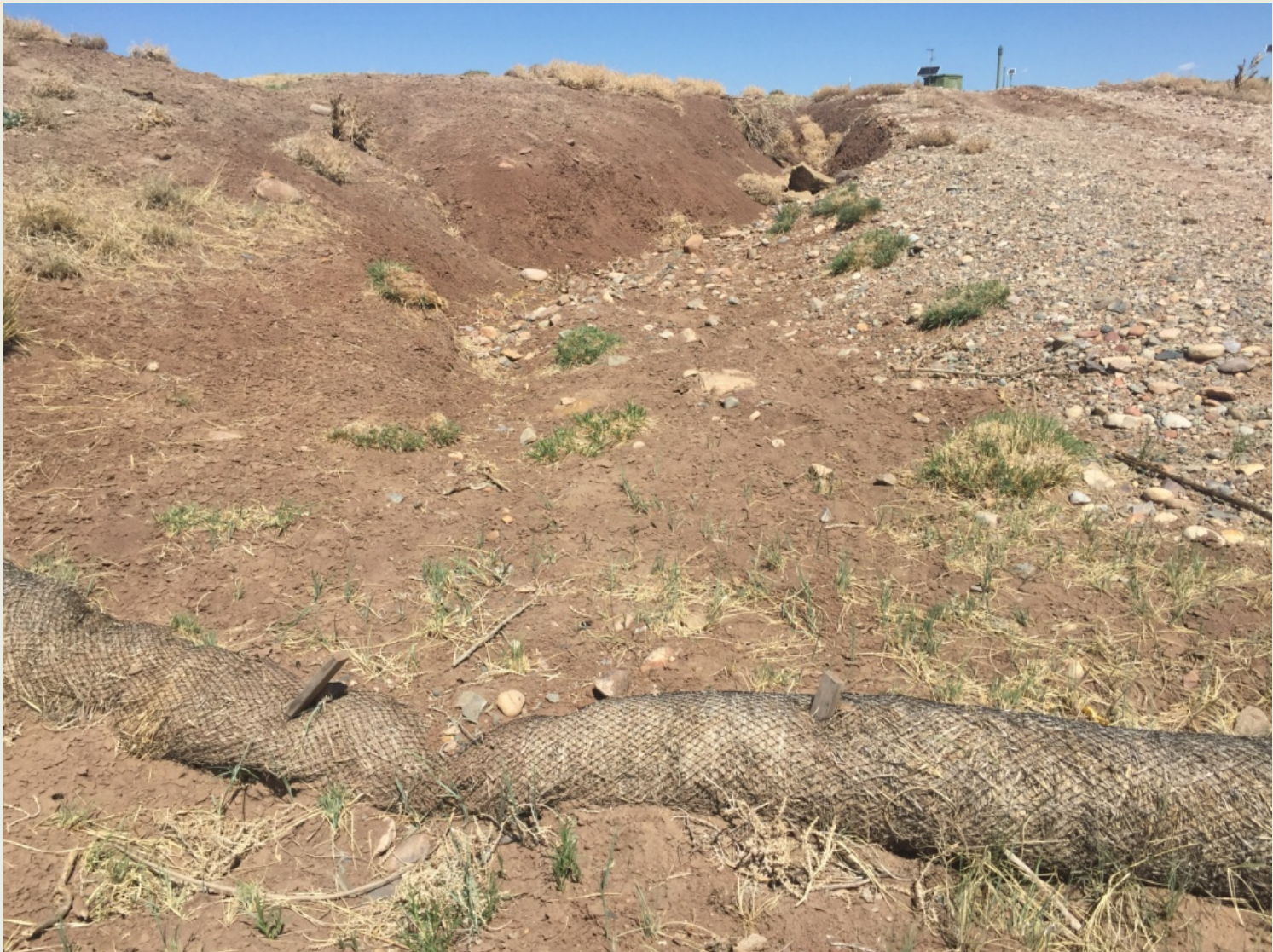
Photo 6. View of eroding channel along northwestern edge of the access road. Slope above channel is not stabilized and is eroding into the channel. Wattle is not sufficient erosion control here and is full of sediment.
