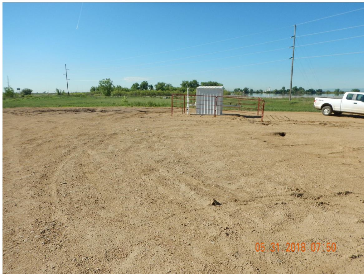
Photo 1. Photo taken from the battery location, facing South. Photo illustrates equipment left on location (meter shed) that needs to be removed. Operator shall conduct final reclamation activities per Rule 1004 by 1/12/2019 and remove equipment ASAP.
