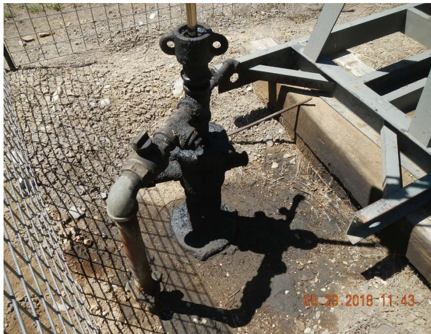
Well head and surrounding soil stained with oil.
