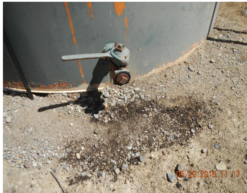
Stained soil beneath load out valve on AST.
