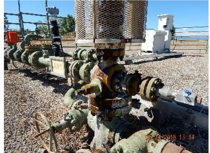
Photo 2: Fluid on wellhead from leaking packing.
